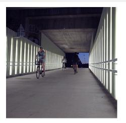
**Produkt:** Tunnel Lighting, Public Space **Material & finish:** Fiberglass-profiles, lit up with LED **Design:** Lightdesign w. Lighting Sweco DK
